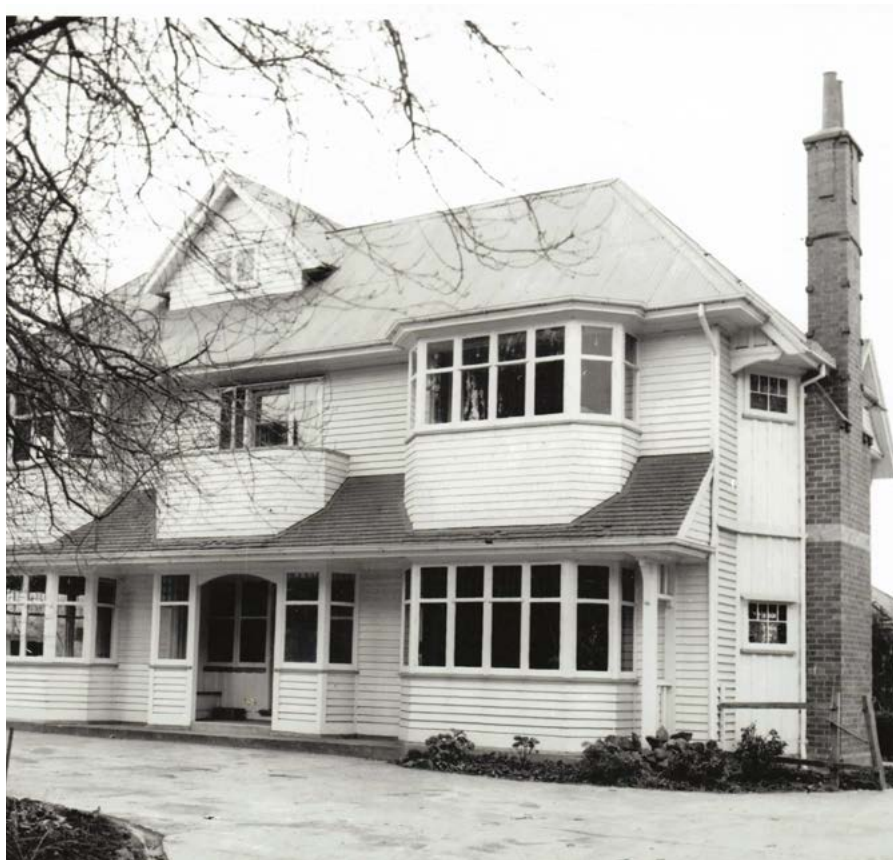
THE HOHEPA CANTERBURY BARRINGTON STREET SITE.
